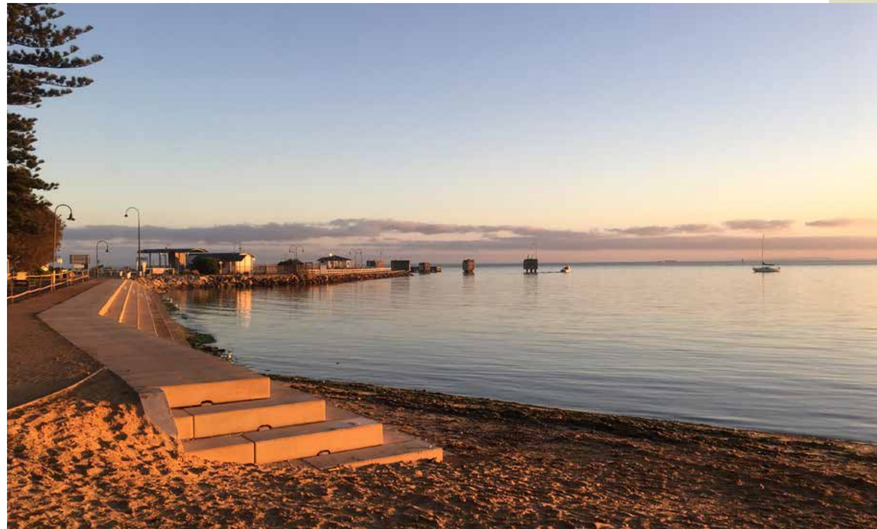
An innovative sea wall at Sorrento demonstrates increased function with seating and viewing opportunities that at the same time minimises impacts of wave energy and protects coastal values. (Maw Civil Marine, Photo: Simon Bulk)
