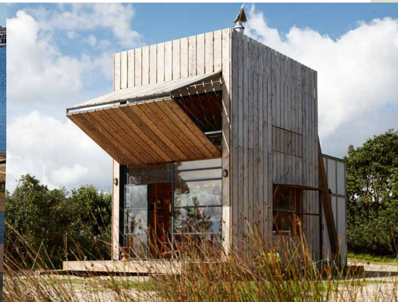
The structure is a compact building featuring sustainable water-saving waste treatment system and flexible screens. It uses ecologically friendly materials and incorporates sustainable, closed-loop systems (a worm tank system to treat waste and two tanks for grey water that can be recycled). When not in use the building is 'boarded up' and blends in amongst the dunes. (The Whanapoua Sled House, Coromandel Peninsula, New Zealand, Photo: Jackie Meiring)
