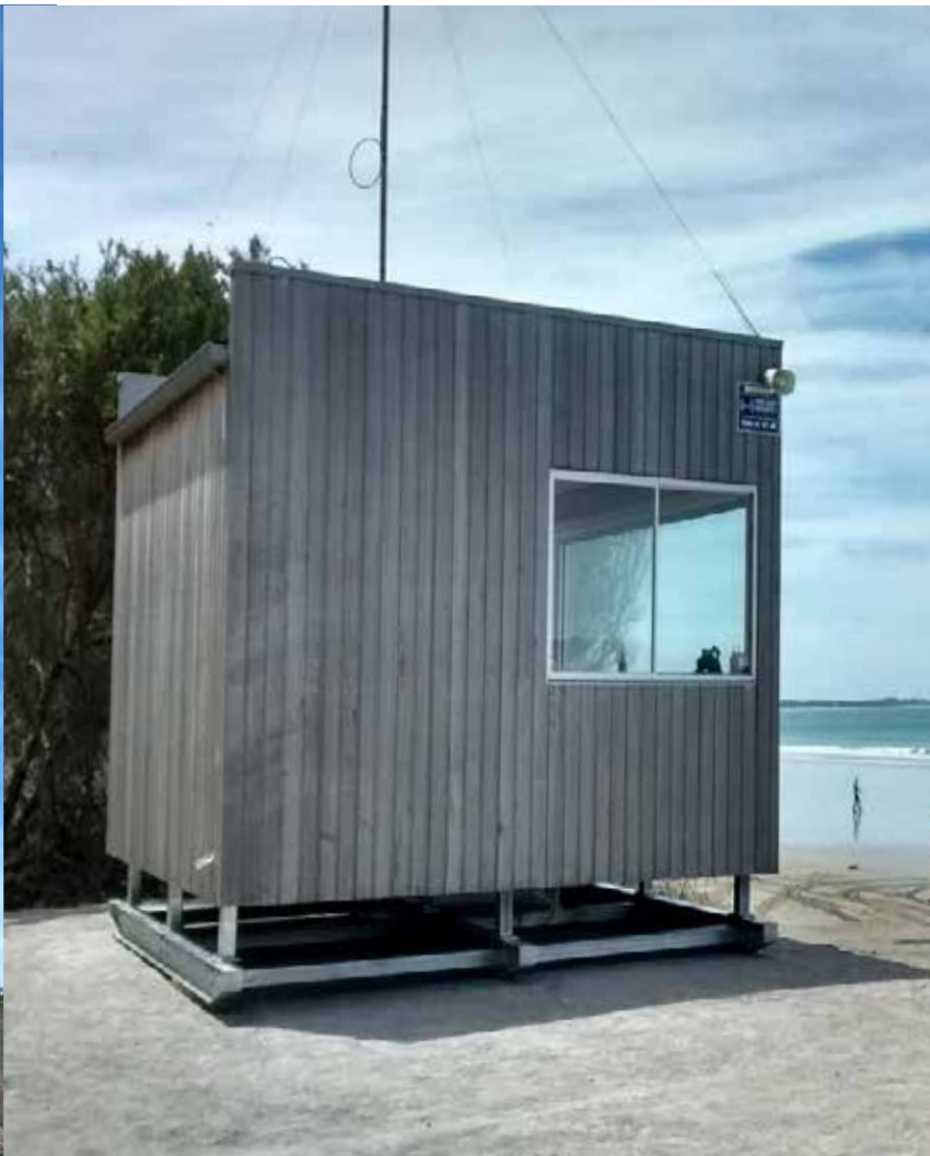
The life-saving club structure minimizes its impact on the primary dune through the setback of the clubhouse behind the dune. A low impact, modular and movable observation structure provides an alternative to hard engineering options with the ability to be moved in response to dynamic natural coastal processes. (Inverloch Surf Life Saving Club, Victoria, Photo: DELWP)
