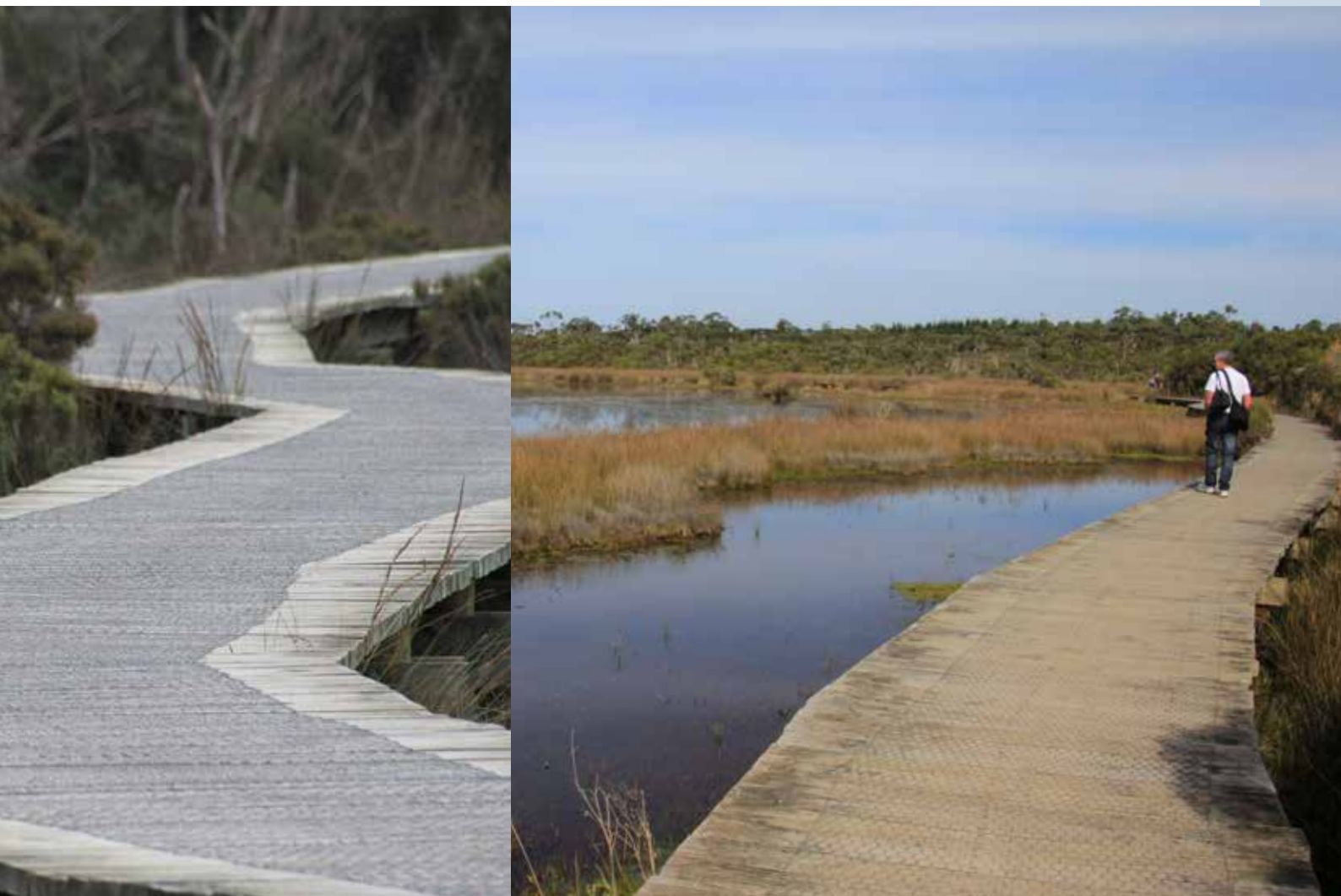
The boardwalk infrastructure accommodates and maintains natural drainage patterns and site vegetation while providing access and viewing opportunities. (Bittern Coastal Wetlands Walk, Hastings, Photos: Katherine Cooper)
