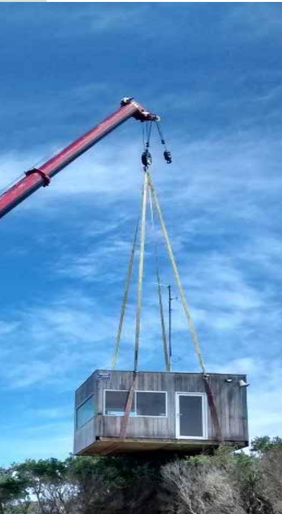
The life-saving club structure minimizes its impact on the primary dune through the setback of the clubhouse behind the dune. A low impact, modular and movable observation structure provides an alternative to hard engineering options with the ability to be moved in response to dynamic natural coastal processes. (Inverloch Surf Life Saving Club, Victoria, Photo: DELWP)
