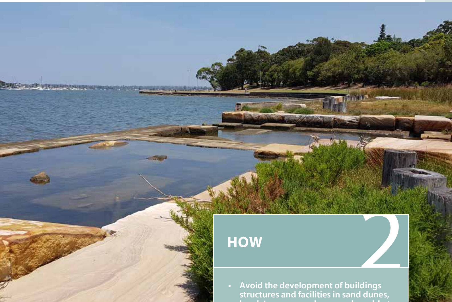
Demonstrates an alternative engineering option for coastal protection rather than a seawall. (Carss Bush Park foreshore, Kogarah Bay NSW Photo: Tom Heath)
