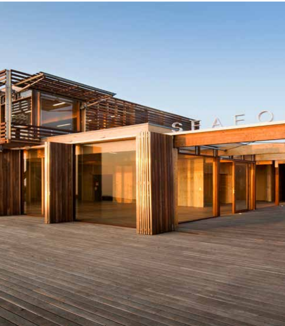
Exposure to wind and solar penetration is managed through careful orientation of building elements. (Seaford Life Saving Club, Seaford, Design: Robert Simeoni Architects, Photo: John Gollings)
