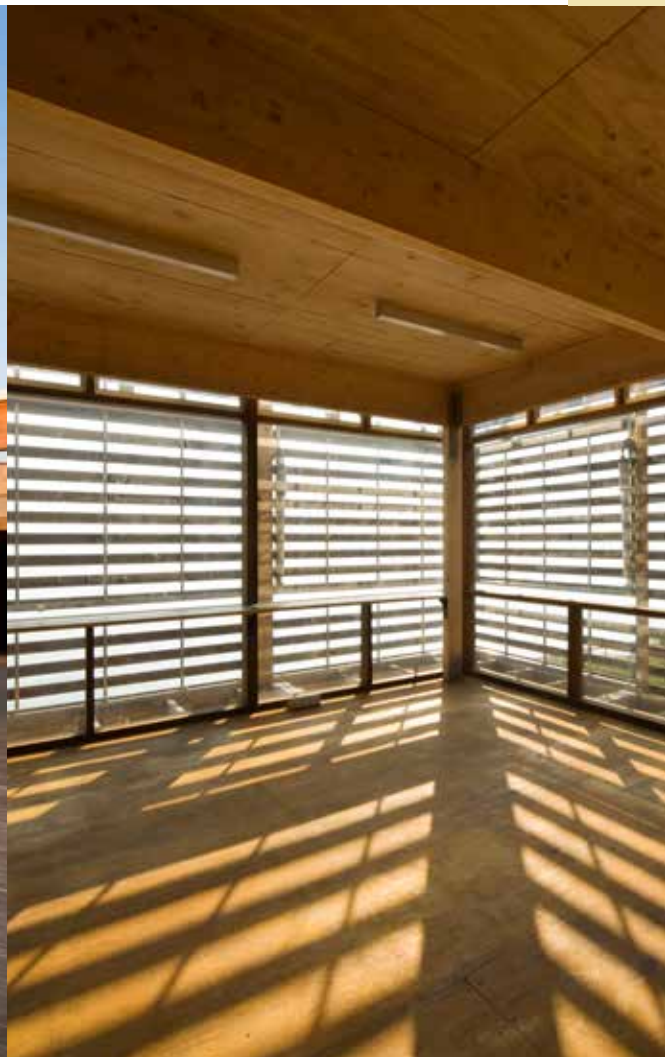
Timber batten screens optimize natural light and facilitate cross ventilation but can be adjusted to provide protection from prevailing winds or shield against summer sun. (Seaford Life Saving Club, Seaford, Design: Robert Simeoni Architects, Photo: John Gollings)
