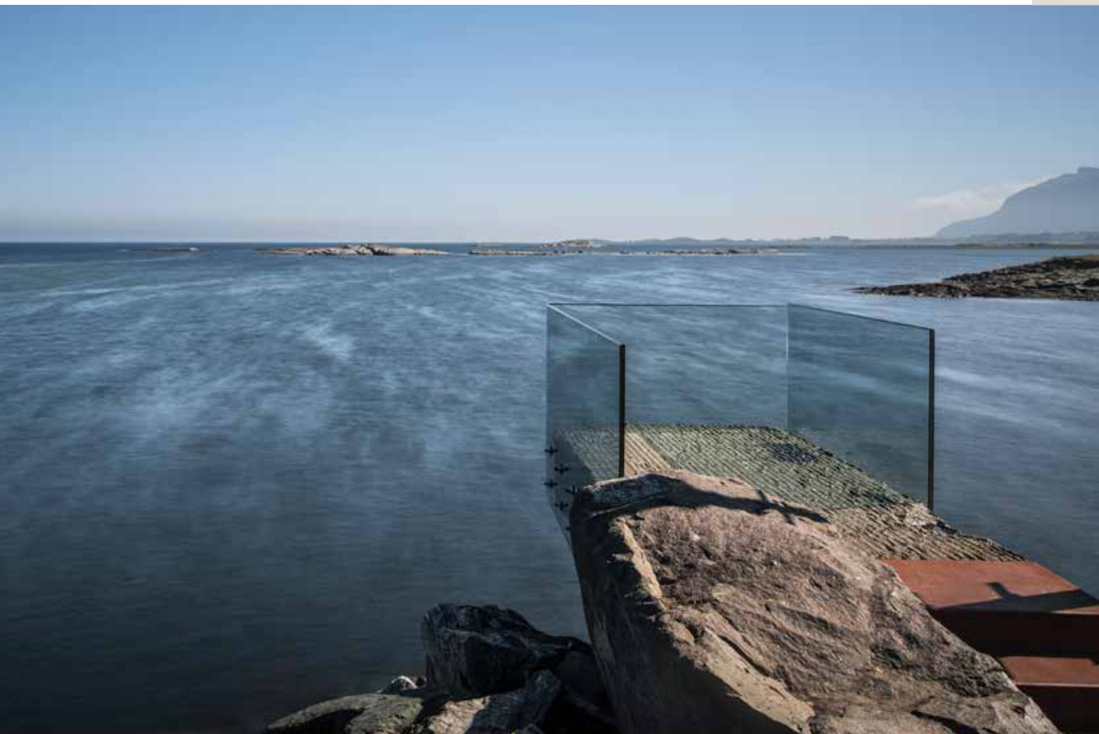
Lookout design uses materials that integrate with the site geology and surrounding landscape. Siting minimizes ground disturbance and maintains natural slope. (The Askvagen Outlook, Norway, Photo: Roger Ellingsen)
